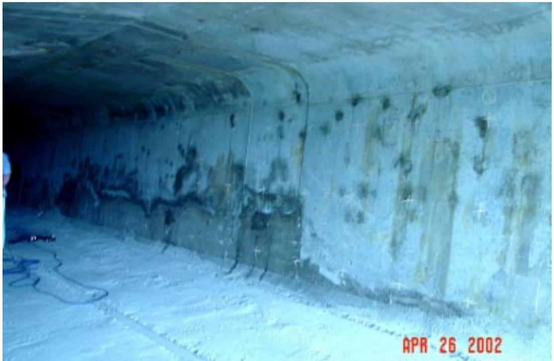
Fig. 5 Repair Patching.
