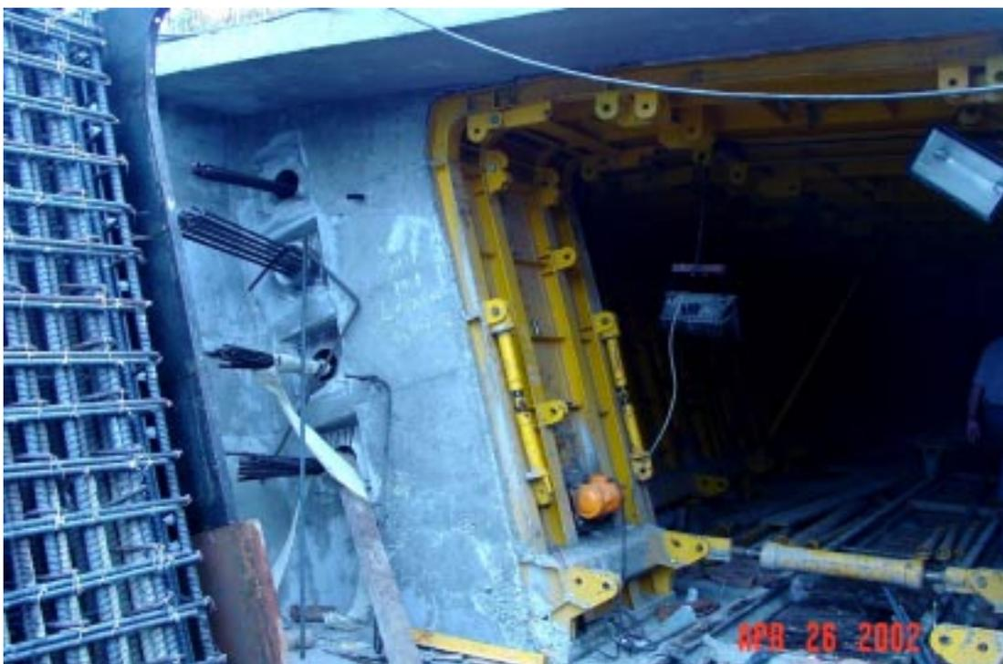
Fig. 4 Post-Tensioning Details at Diaphragm.
