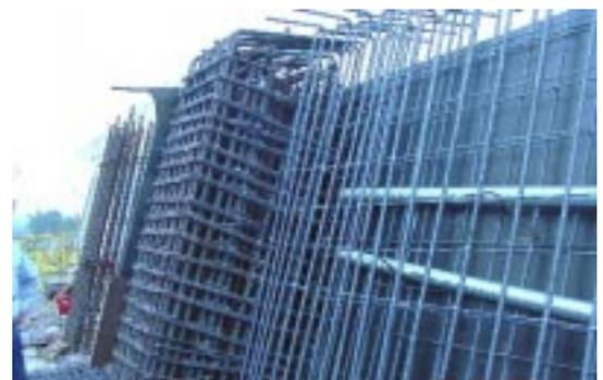
Fig. 6 Density of Steel Reinforcement.
