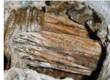
Condition of duct
