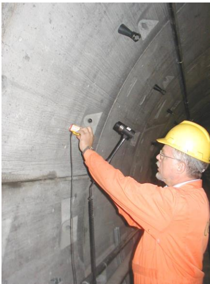
Testing for voids behind tunnel lining
