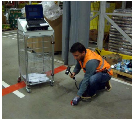
Testing for voids below industrial floor slab
