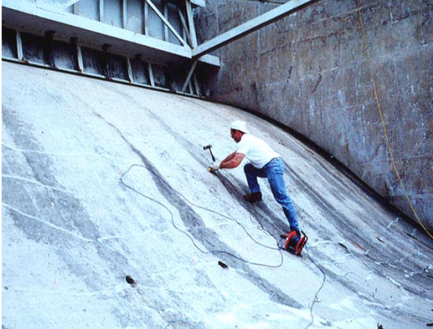
Testing for delaminations in dam spillway
