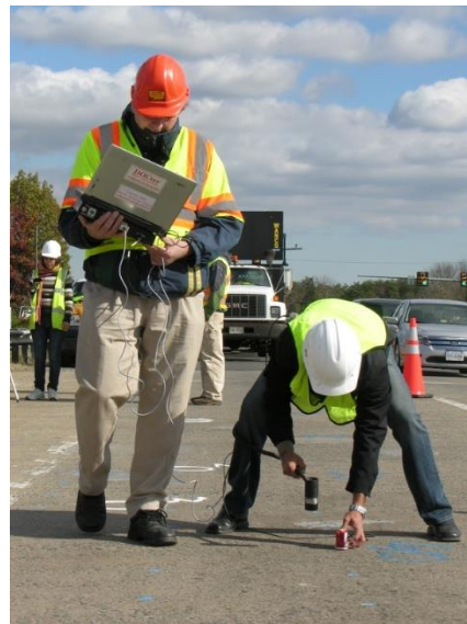
Testing for delaminations in bridge deck
