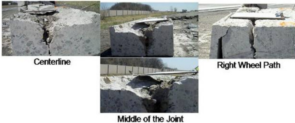
Figure 13. Forensic sample sections used to verify the concrete condition on the underside at various locations near the transverse joint.
