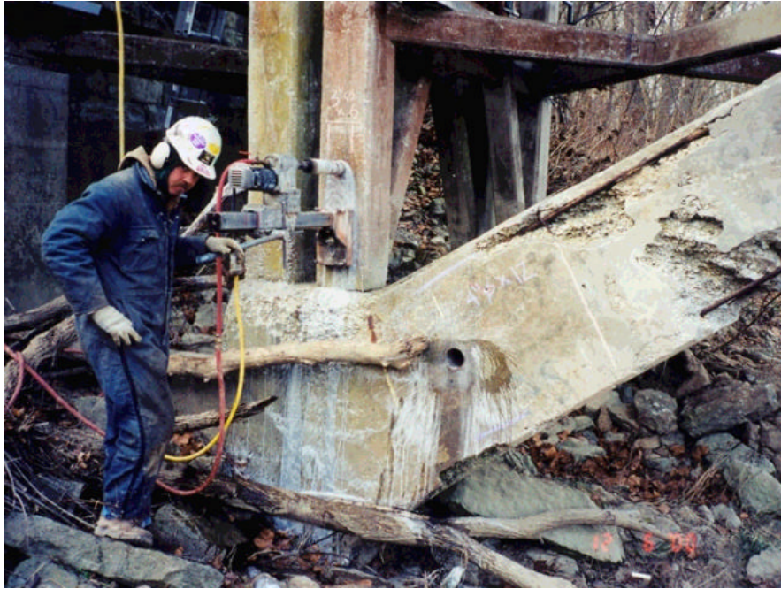
Figure 9. Coring Operation
