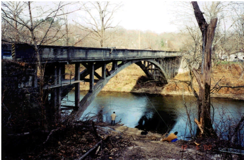
Figure 8. Putnam County Bridge
