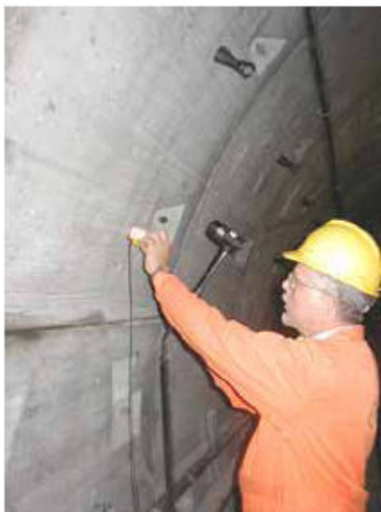
Testing for voids behind tunnel lining
