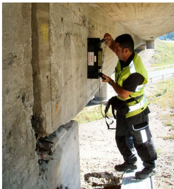
Scanning along web
