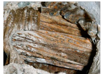
Condition of duct
