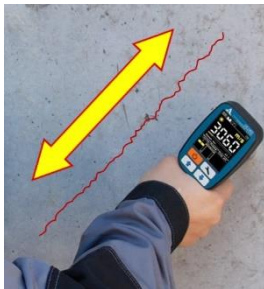
Measure transit time ( t_p ) parallel to crack
