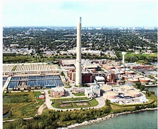
Figure 6. Ashbridges Bay Chimney
