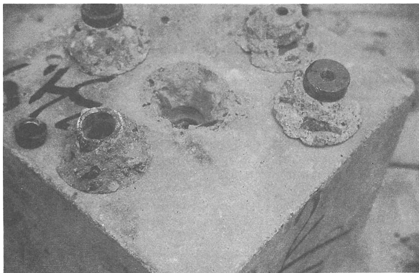
Figure 51. pull-out testing by LOK-test and CAPO-test carried out on a 200 mm concrete test cube.
