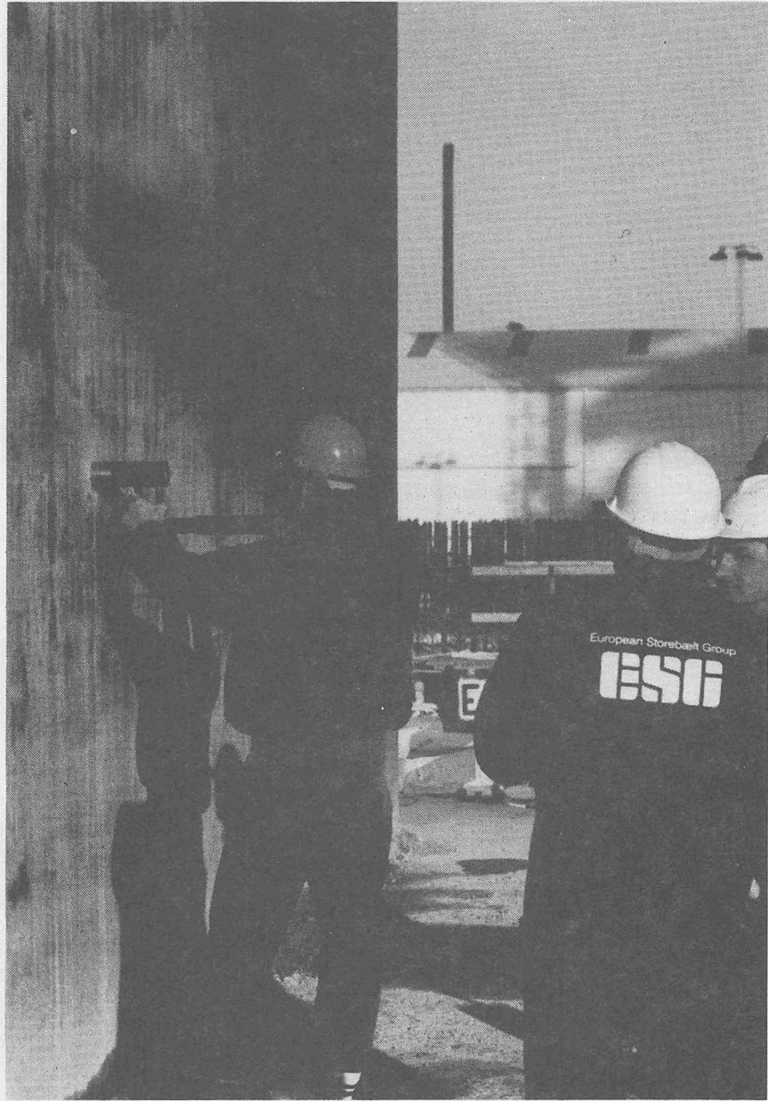
Figure 36. Testing of a caisson by CAPO-test at the final examination.
