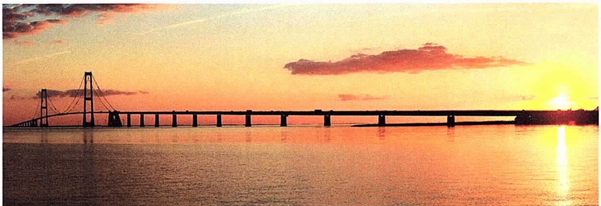
Fig. 4. Panoramic of the East Bridge.
