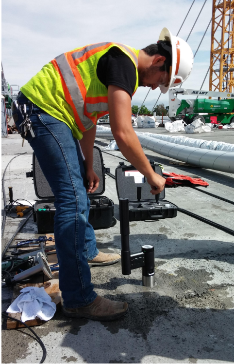
Joints at Ohio River Bridge, Louisville, Kentucky, USA being tested for compressive strength with CAPO-TEST
