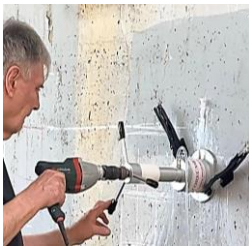
Preparation for the BOND-TEST, coring around the disc glued on prepared surface
