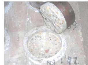
Tensile failure of the concrete. Max pullforce registered and divided by the area to get the MPa's
