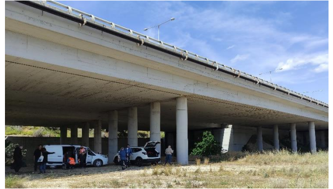
...and the bridge B044 close to the Corinth Canal, Peloponnese, Greece
