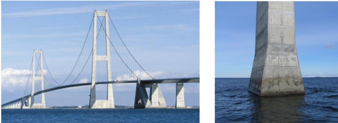
Figure 30. The Great Belt Link's suspension bridge and one of its piers selected for testing for service life. The pier was constructed using plywood form kept on for 3-5 days before stripping. LOK-TEST performed met the requirements.
