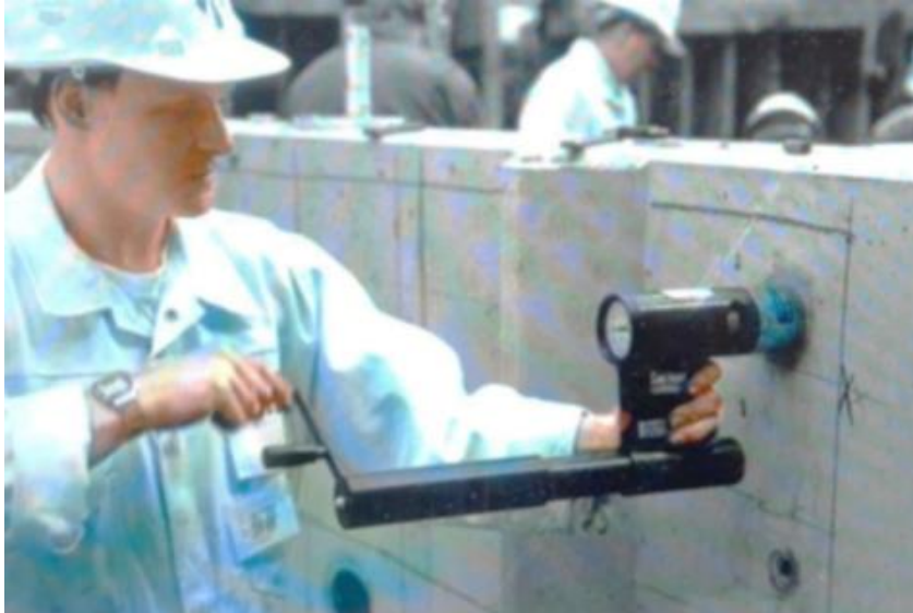
Figure 42. CAPO-TEST in progress. Three CAPO-TESTs in each quarantined element were performed.
