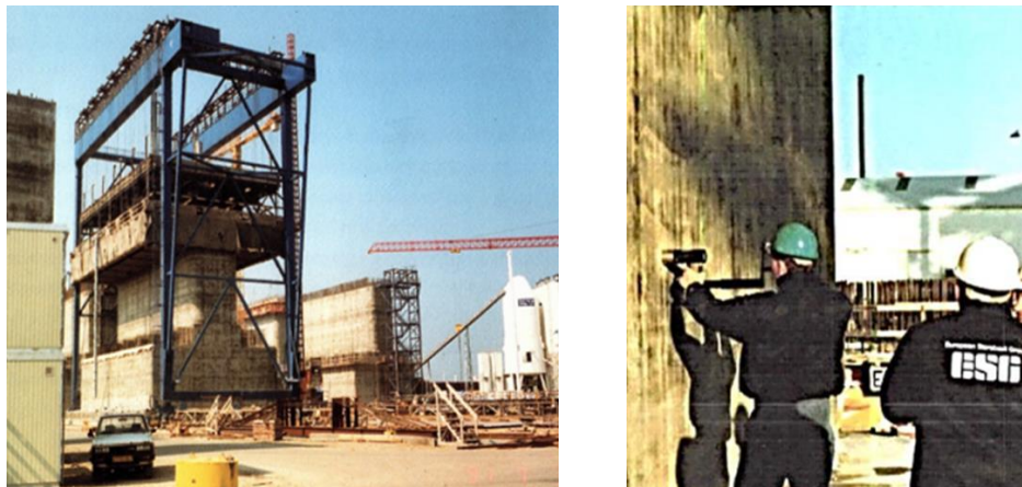
Figure 27. Steel slipform used for the caissons (left), and CAPO-Testing (right).
