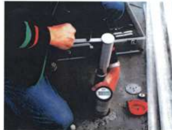
Figure 1: The Lok-test jack in position.
