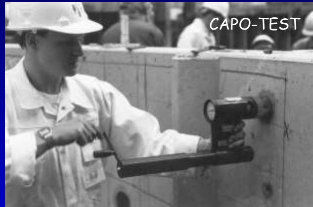
Translink, UK, Residual strength of tunnel segments
