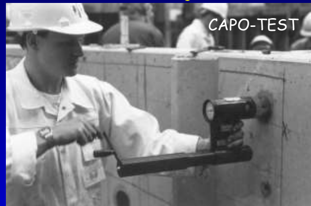
Translink, UK, Residual strength of tunnel segments
