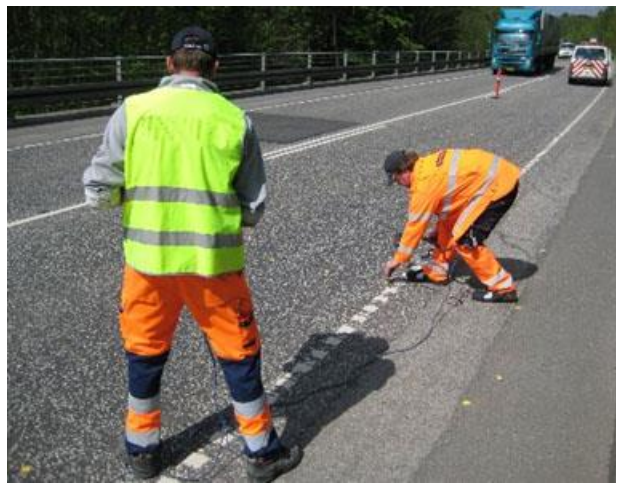
Testing for delaminations in asphalt covered concrete pavement
