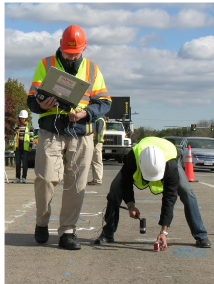
Testing for delaminations in bridge deck
