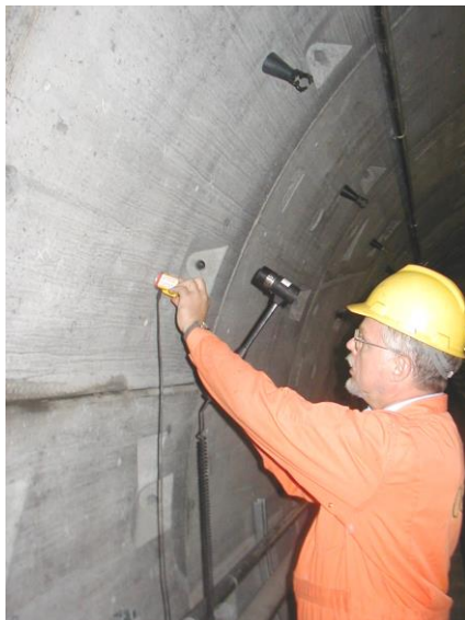
Testing for voids behind tunnel lining
