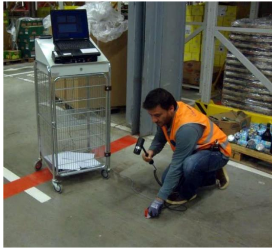
Testing for voids below industrial floor
