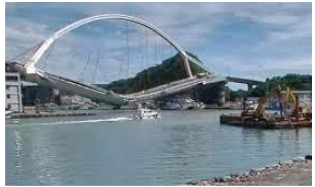
More bridge collapses caused by corrosion of cable duct strands, Italy & Taiwan
