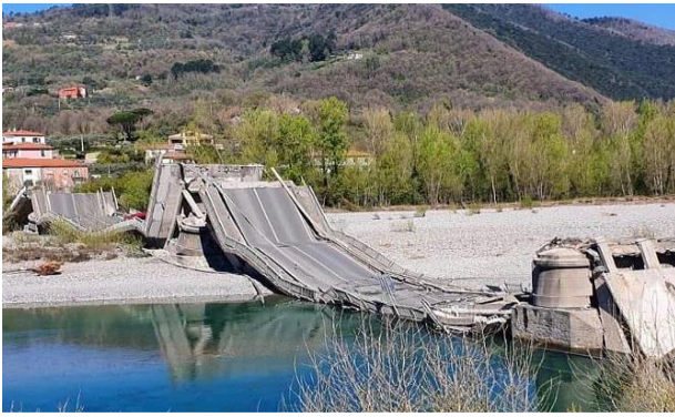
More bridge collapses caused by corrosion of cable duct strands, Italy & Taiwan
