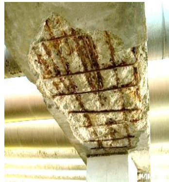
Reinforcement corrosion caused by chlorides/carbonation and bad cover layers, Middle East, Norway and USA
