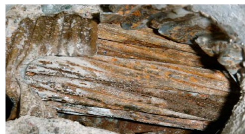
Corroded strands in an empty steel duct
