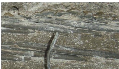
Sound strands in well injected duct
