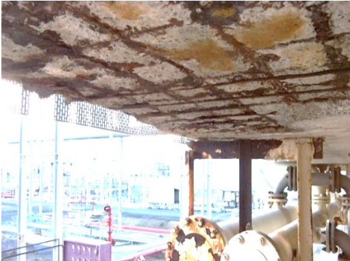
Reinforcement corrosion caused by chlorides/carbonation and bad cover layers, Middle East, Norway and USA
