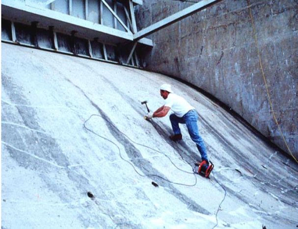
Testing for delaminations in dam spillway
