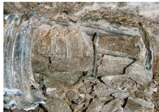
B-scan at location (2) with no voids indicated in grouted duct. The excavation reveals the strands encased with grout; some of it was fractured in the process and this exposed some wires.
